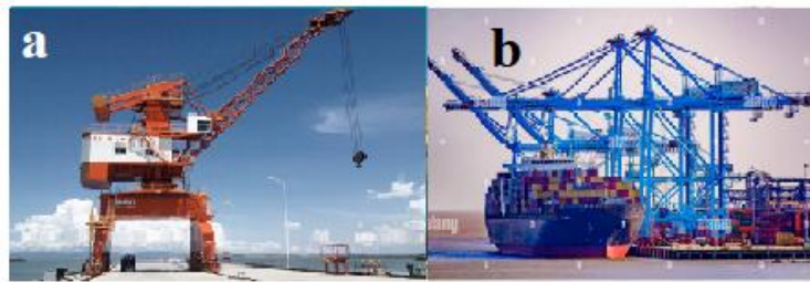
Fig. 3. Port cargo handling equipment: a – gantry crane; b – container handling system.
