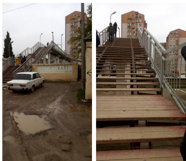
Fig. 2. Current state of the crossing at the Khirdalan passenger station.
